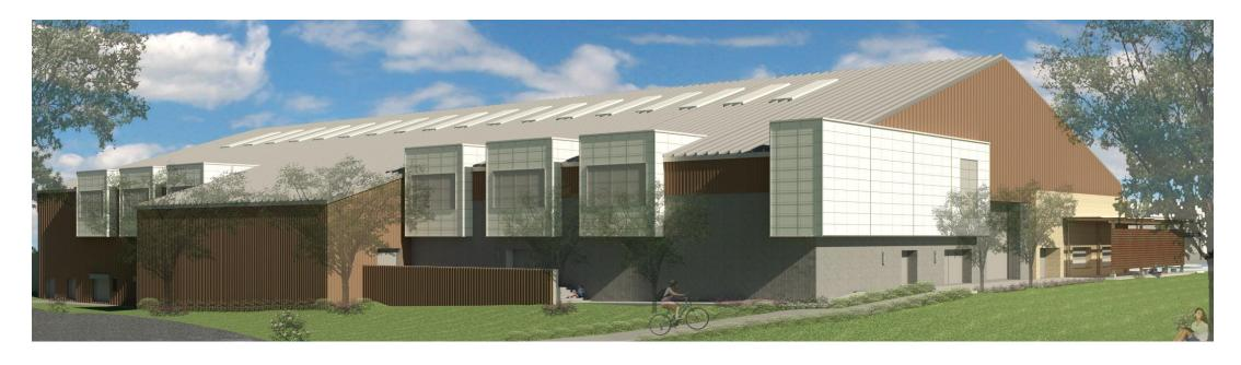
New Exterior finishes \* New roof profile \* New Roof Panels \* Upgrade dressing rooms, showers & restrooms \* New tile at pool surface area \* Refurbish diving platforms \* New LED lighting \* New Fire Sprinkler System \* New interior finishes
